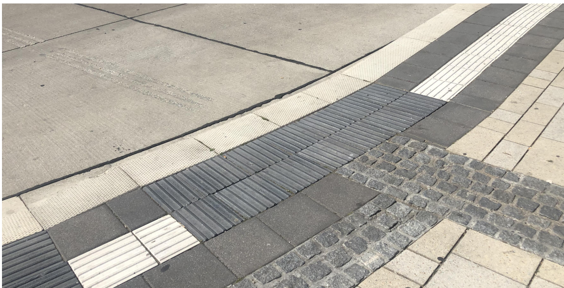
Figure 1.2: Tactile pavings in an urban environment near a bus stop. The different grooves in the stone indicate the walking directions. Little bumps on the curb limit the walkway.
