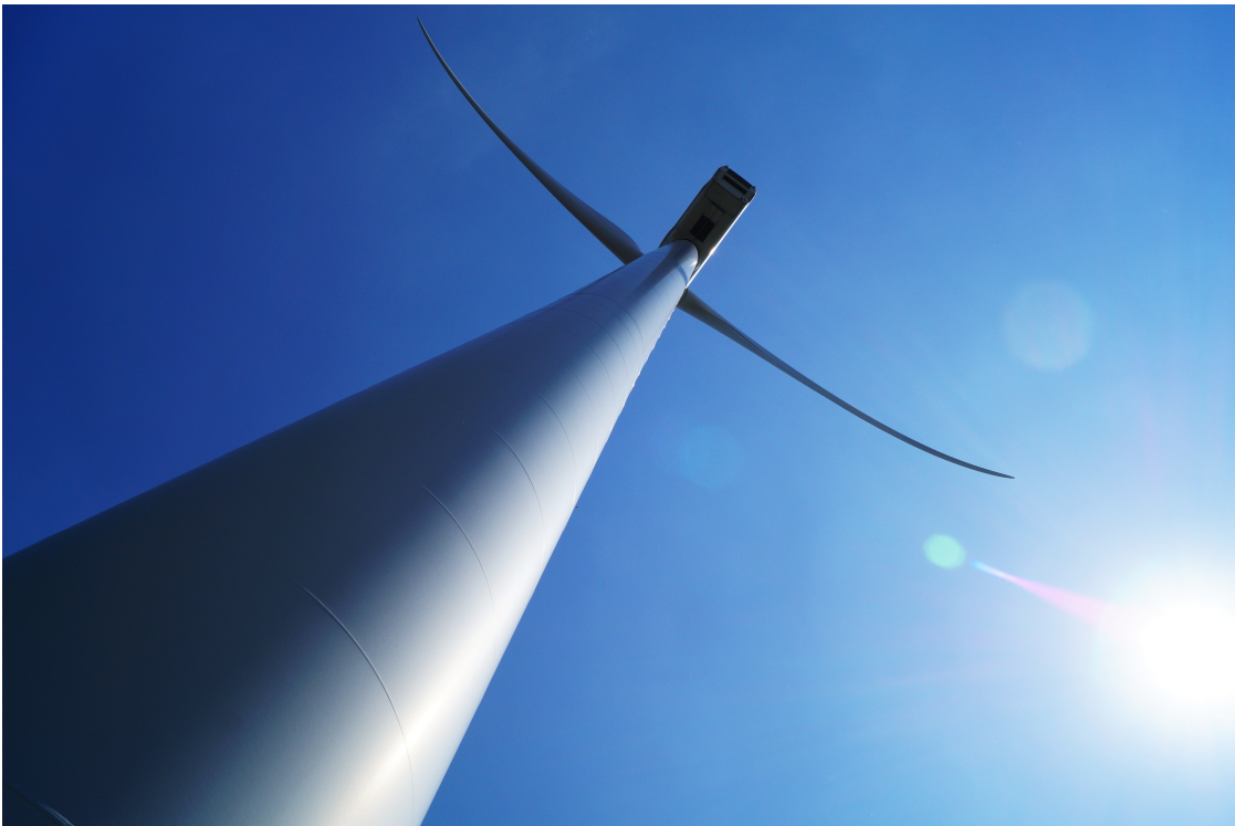
Figure 1-2.: Wind turbine subject to seemingly large blade deflections.
