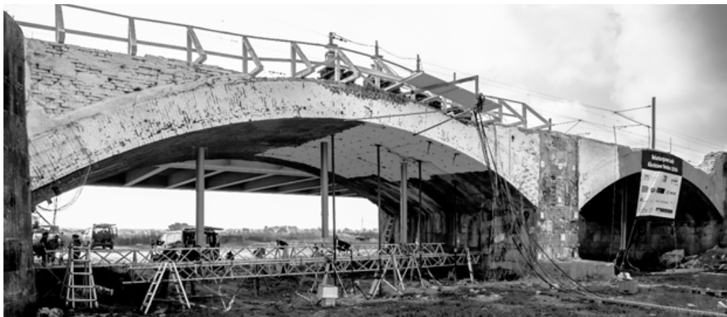
Figure 2. Side view from west of the arch 4 of the historic masonry arch bridge. The whitewashed area indicates the area of the direct influence of the load application. On the bridge: four hydraulic cylinders for the load application (Paffenholz et al. [27]). Reproduced with permission from Paffenholz, AVN; published by Wichmann-Verlag, 2018.
