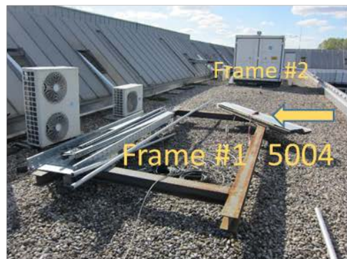
5004: T-Beam Base Frame #1 (top of steel T-beam frame at corner, see sketch)
