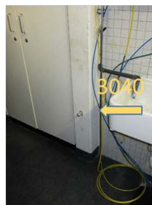
3040: Wall marker (bolt) (Lab C0.40)
