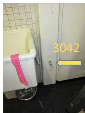
3042: Wall marker (bolt) (Lab D0.42)
