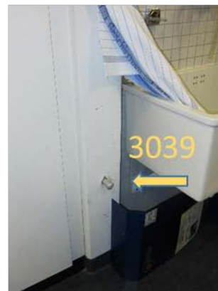
3039: Wall marker (bolt) (Lab D0.39)
