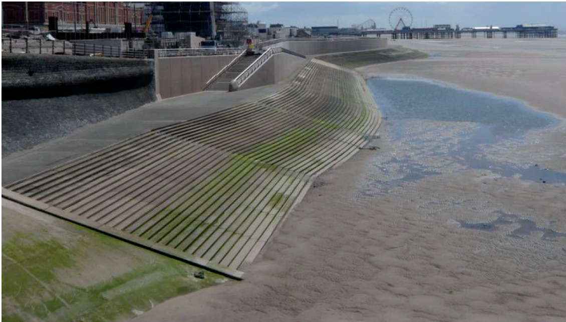
Figure 2.2: Significant algae growth on the Blackpool revetment visible at low tide (photo taken from Rowe (2012a)).
