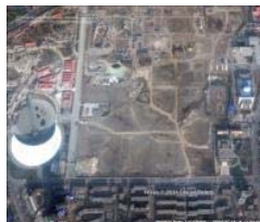
Figure 46b: Constructing Cultural Park in 2009 (Map data: Google, Digital Globe)
