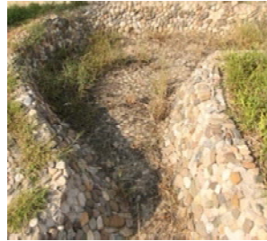
Figure 89a: Shallow ditch
