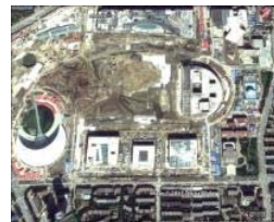
Figure 46c: Constructing Cultural Park in 2011 (Map data: Google, Digital Globe)
