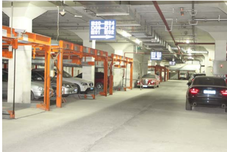
Figure 90: Garage underneath the artificial lake
