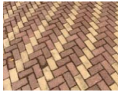
Figure 92b: Pavement II
