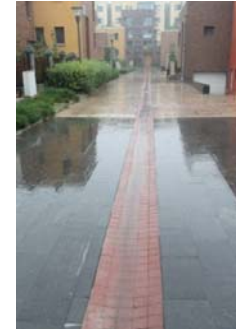
Figure 33: Drainage using gradient on a secondary road
