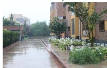
Figure 38: Open gutter in secondary road connected to central waterscape
