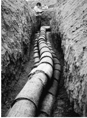
Figure 1: Three different pipes of variable diameter combined together were used as water conveyance lines
