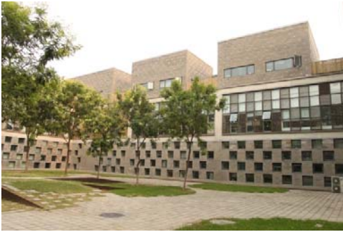
Figure 70a: Pavement and building surface in the yard
