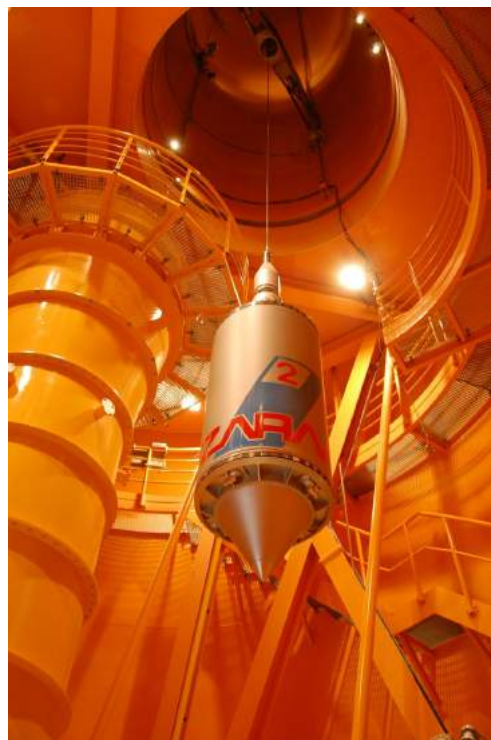
Figure 34: The capsule being hoisted to the top of the drop tube prior to first drop. The deceleration container is visible on the left.
