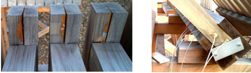
Figure 8. Left: accelerated L-joint test. Mortise shows cracks. Right: embedded test with open mortise.
