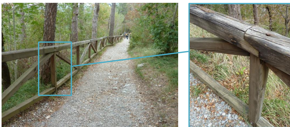
Figure 2: Handrail in 'Škocjanske jame' national park, Slovenia. Different exposures, varying from UC 4 (posts) to UC 3.1 (stabilizer and handrail). In addition, water trapping is caused by lap-joint-construction of segmented handrail (UC 3.2).
