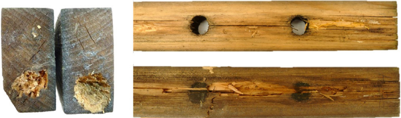
Fig. 3: Brown rot decay starting from water traps at contact faces between end grain and end grain (left) and between side-grain and side grain (right)
