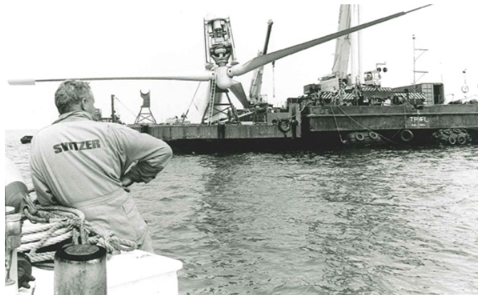
Figure 1.1: Turbine installation at Vindeby Offshore Wind Farm 1 .
