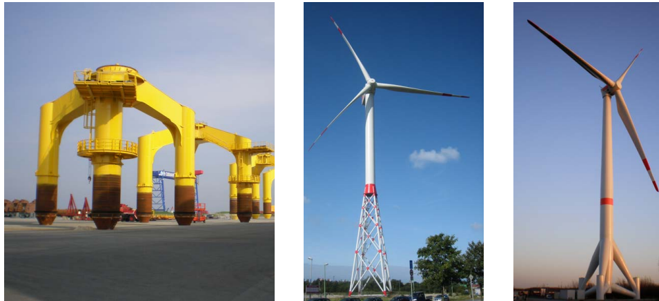
Figure 2.12: Branched support structures for a water depth of approximately 30 m. From left to right: Tripiles at construction site, jacket and tripod installed onshore (pictures: private).
