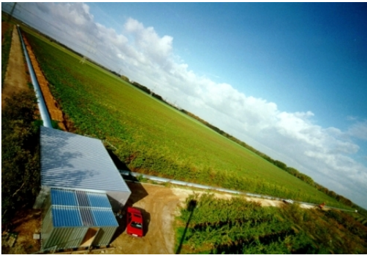
Figure 1.8: GEO600 detector, with an armlength of 600 m, located at Sarstedt near Hannover, Germany.
