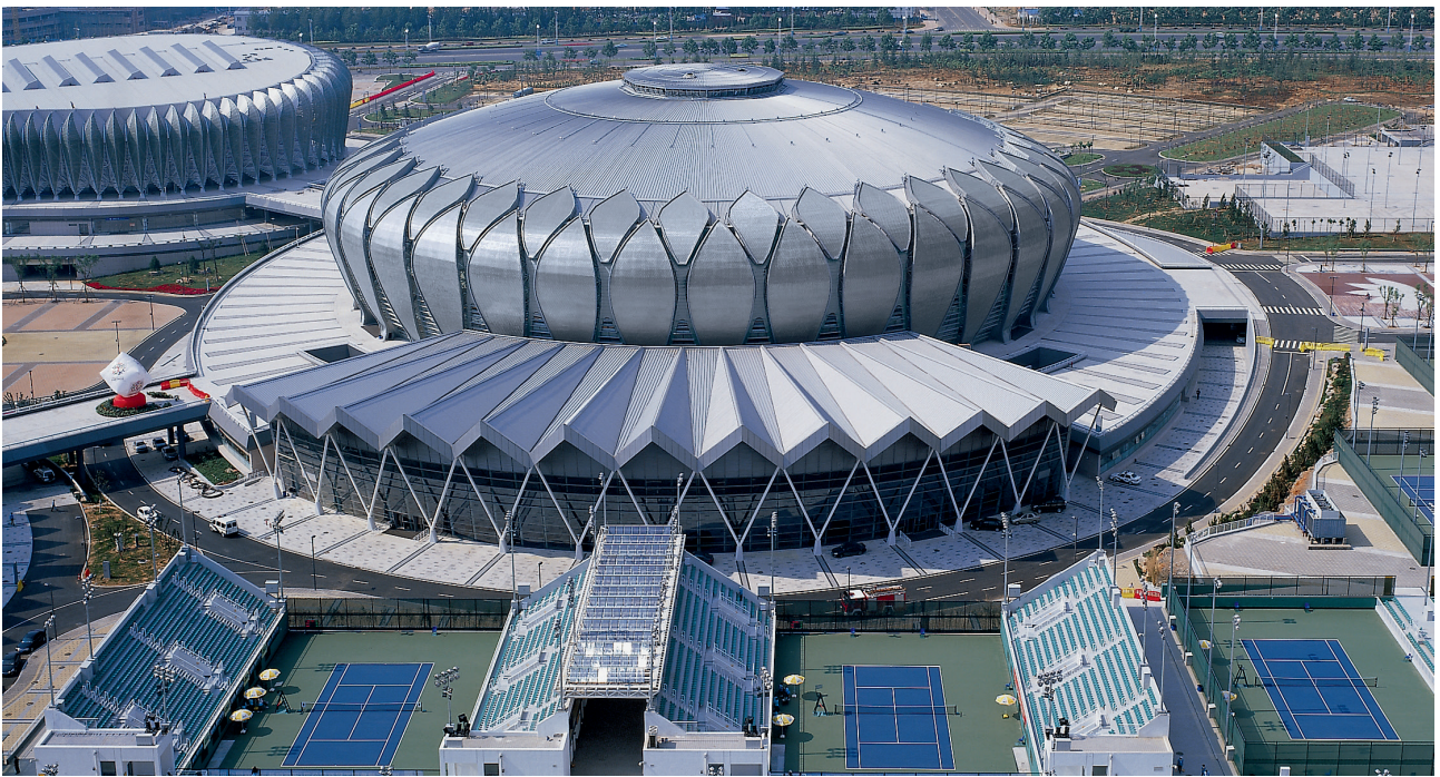
Abbildung 4: Olympic Sports Centre, Jinan, China. Architekt: China Construction (Shenzhen) Design International, Shenzhen, China. © Rheinzink.
