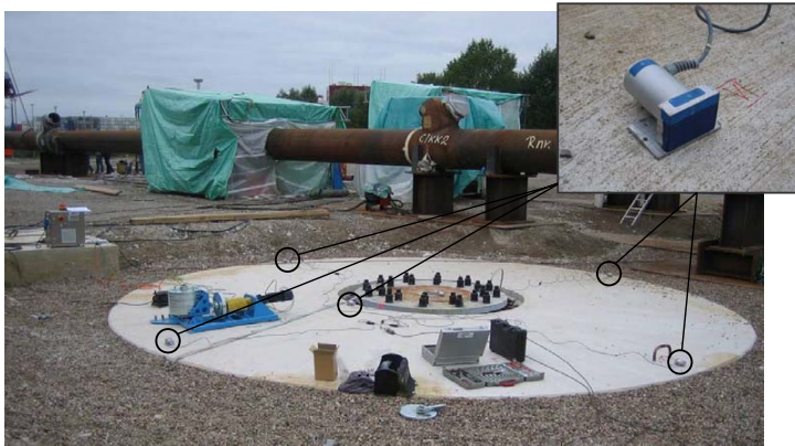
Measurement setup for the single foundation body and geophone
