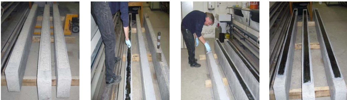
Figure 3-4: Strengthening concrete beams with CFRP
