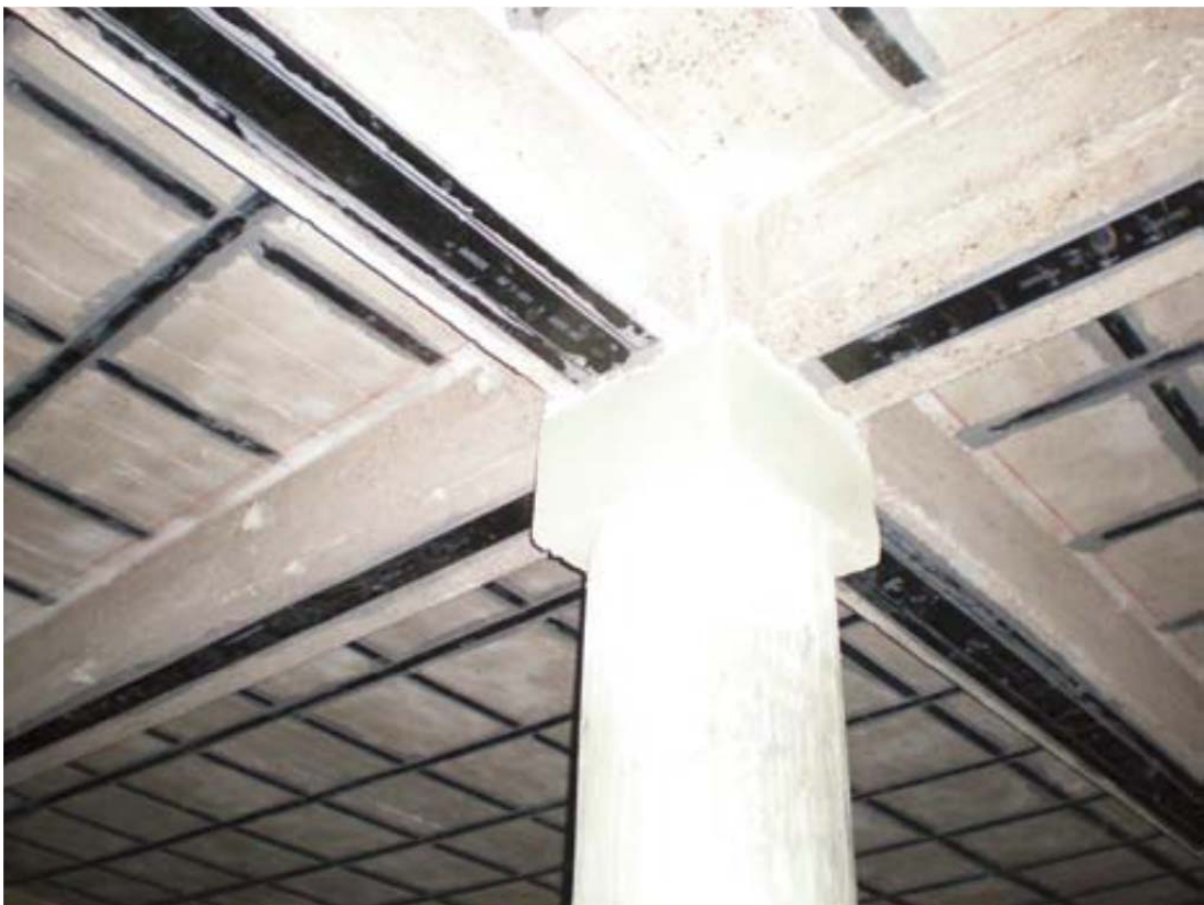
Figure 2-1: Reinforced concrete beams and slabs strengthened with FRPs ( (Amélie Grésille, 2009)
