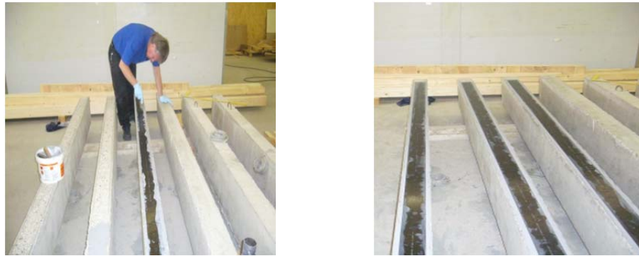
Figure 3-9: Strengthening concrete beams with CFRP
