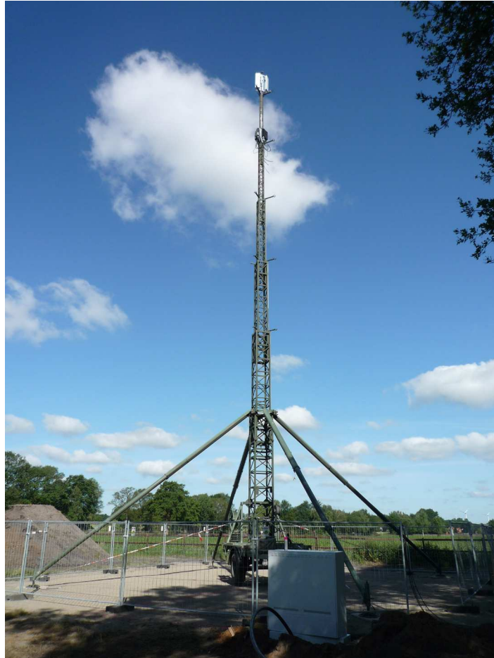
Figure 6: WiMAX base station tower of height 25 m erected in Hetzwege
