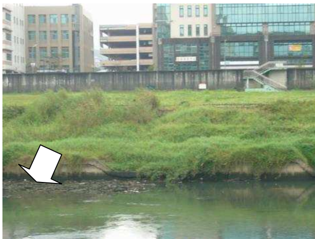
Location: at the right side of Nanhu riverside park (L1040502)
