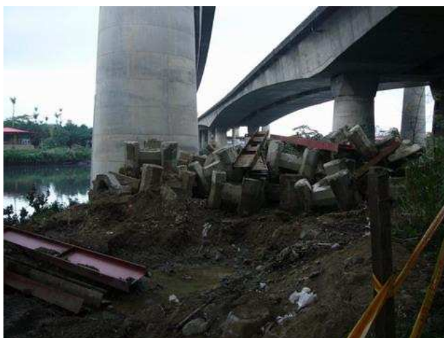
Location: under the Zhongshan Bridge (L1040838)
