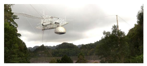
**Figure 3.1:** View of the Arecibo telescope from the terrace in front of the control room facing South. The 305-m dish is at the bottom of the photograph, the western tower can be seen on the right, the eastern tower on the left behind the trees (the northern tower is on top of the hill to the left). Left of the middle, the platform with the 430-MHz line feed and the Gregorian dome housing the ALFA receiver is visible.
