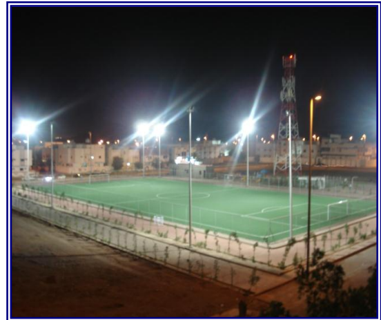
Figure no. (4.1.50) night view of plaza
