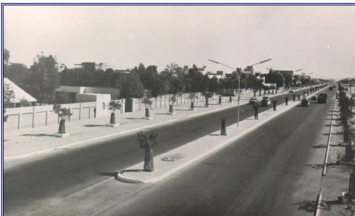
Figure no. (4.2.19) A view of one of Jeddah's streets in the early Saudi period
