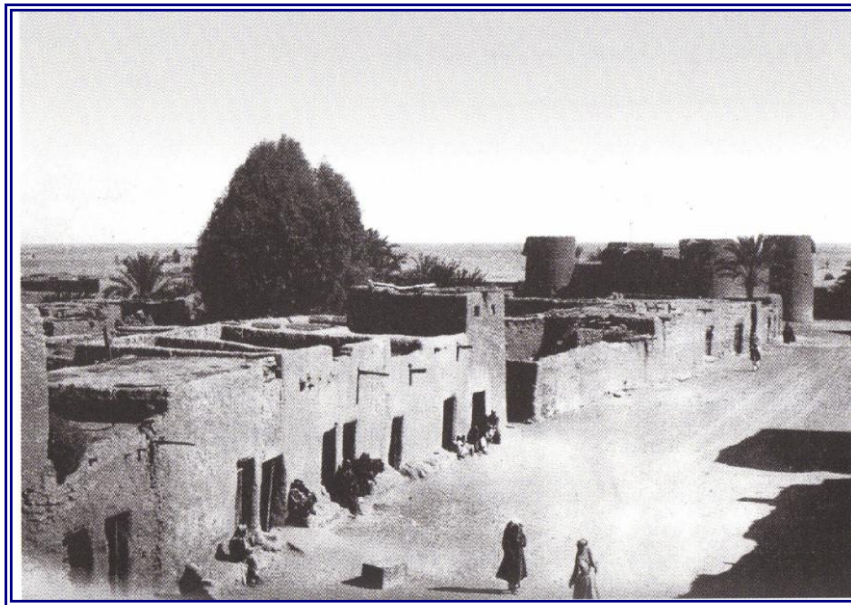
Figure no. (4.3.8) View of Tabuk city's main road and some residences in 1957
