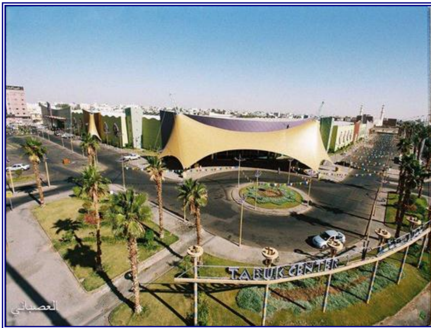
Figure no. (4.3.11) View of a shopping center in Tabuk
