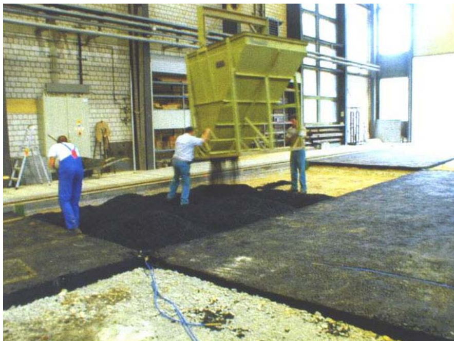
Construction of the asphalt layer in the field no. 2.1 [9]
