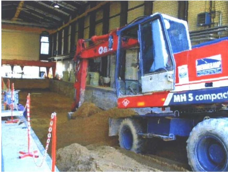
Construction of the gravel ramp in the field no. 3.1 and 3.2 [9]
