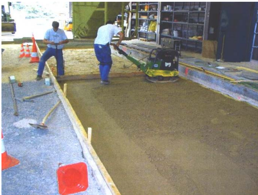
Construction of the hydraulically bound layer in the field no. 1.1 [9]
