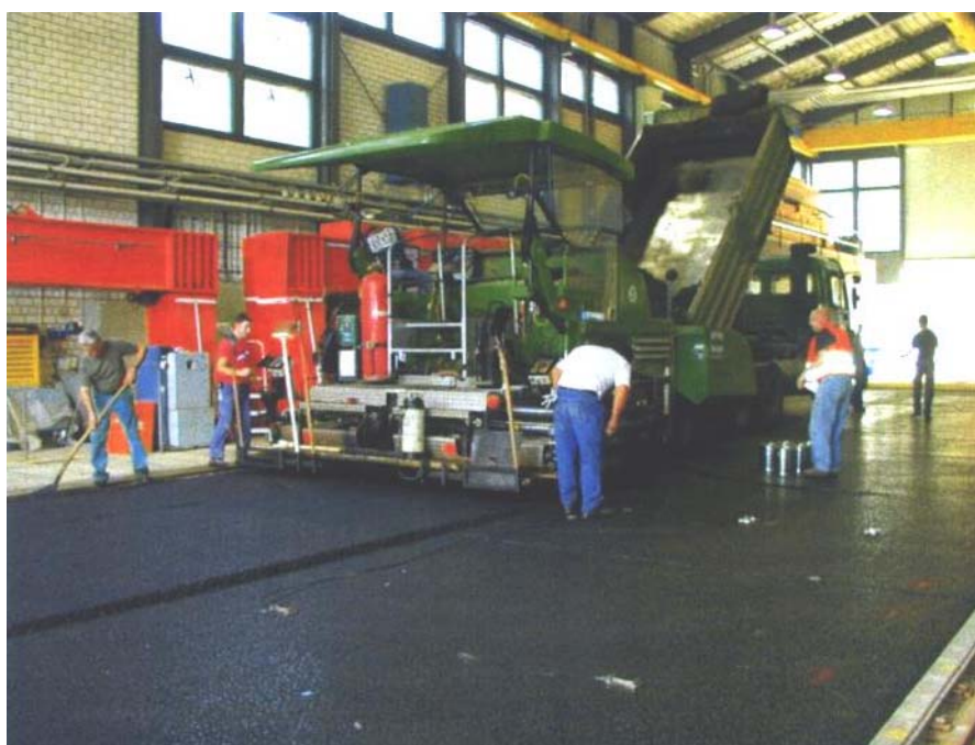
Construction of the asphalt wearing course [9]
