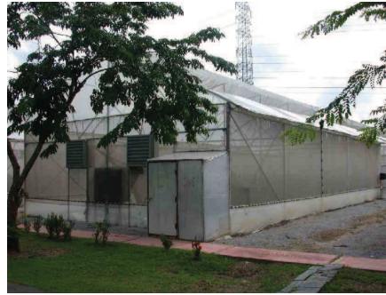
Figure 3.1: Main entrance side of the net-house located at the campus of the Asian Institute of Technology (AIT) in Bangkok, Thailand.
