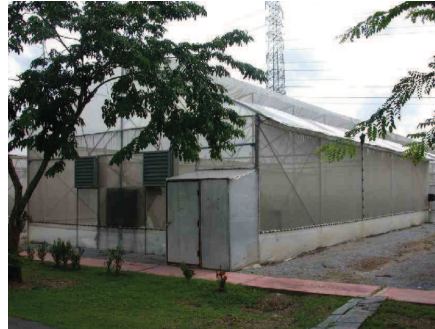
Figure 4.1: Closed net-house located at the campus of the Asian Institute of Technology (AIT) in Bangkok, Thailand.
