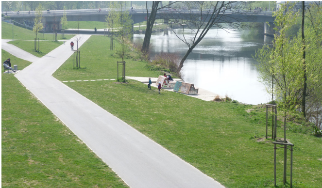
Fig. 2. The Reconstruction of the Benno-Ohnesorg-Bridge with the Newly Designed Ihme Embankment. (DEPARTMENT ENVIRONMENT AND URBAN GREENSPACE, STATE CAPITAL HANNOVER)
