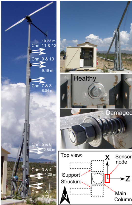
Figure 7.1: The LANL wind turbine.
