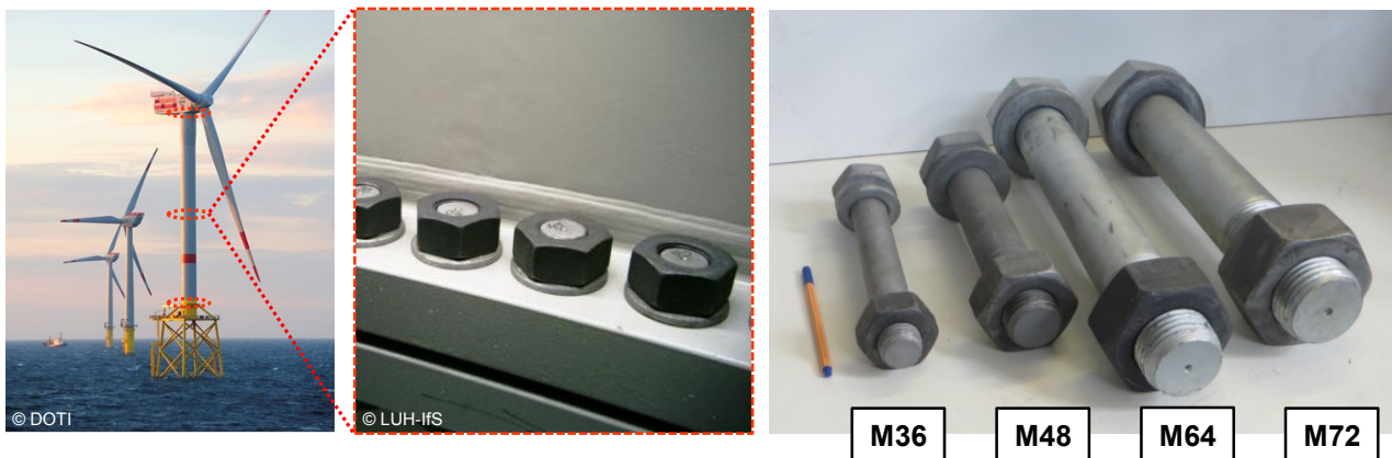
Figure 1-1: Ring-flange connection in wind turbine support structure (left) and HV-bolt sets with large diameters (right)
