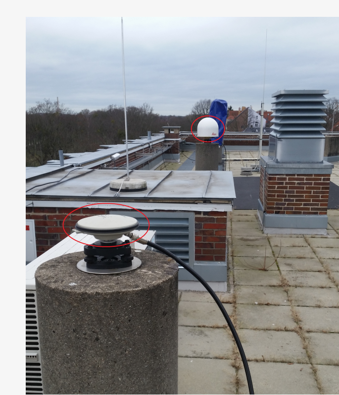
Figure 6: Experimental setup on the rooftop from GIH
