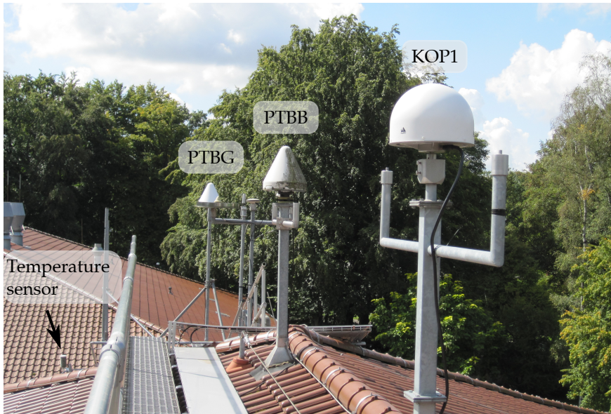
Figure 19: GNSS installations on the rooftop of the Kopfermann building at PTB.
