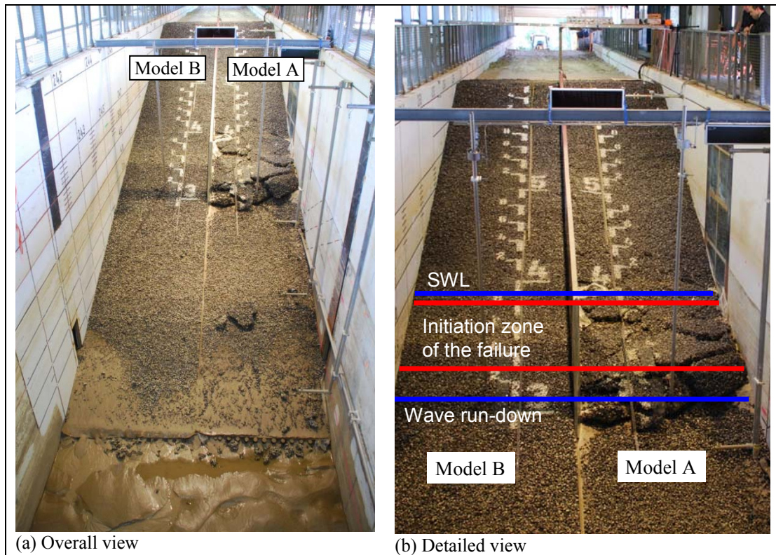
Figure 8. Extent of damage for revetment Model A after regular wave test 09051802 with H = 1.3\text{m} , T = 5.0\text{s} and h = 3.9\text{m}
