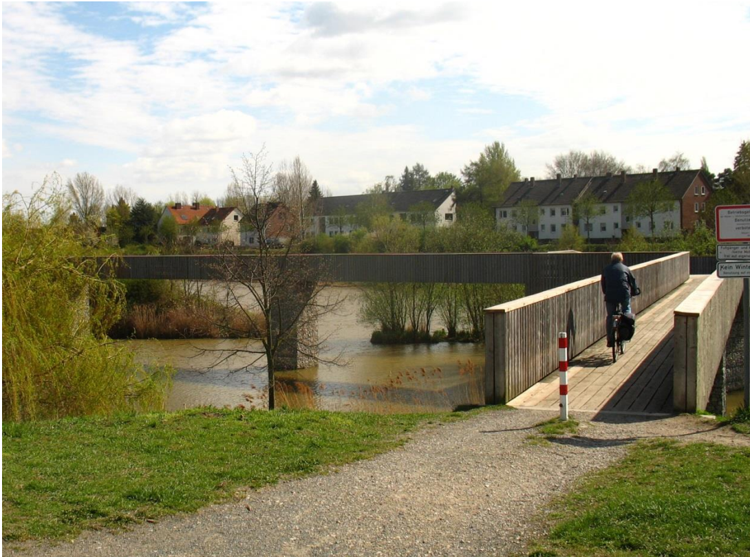
Figure 1 (©Martin Prominski): A bulge or small bay has been created on the edge of the Mittelland Canal (in the background) at the Buchholz Arc in Hannover. The bulge, a habitat with over-average biodiversity, is spanned by a walkable sculpture, which is connected to the local path network.
