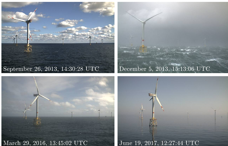
Figure 1.2: Offshore wind turbines of the offshore wind park alpha ventus ©FuE-Zentrum FH Kiel GmbH
