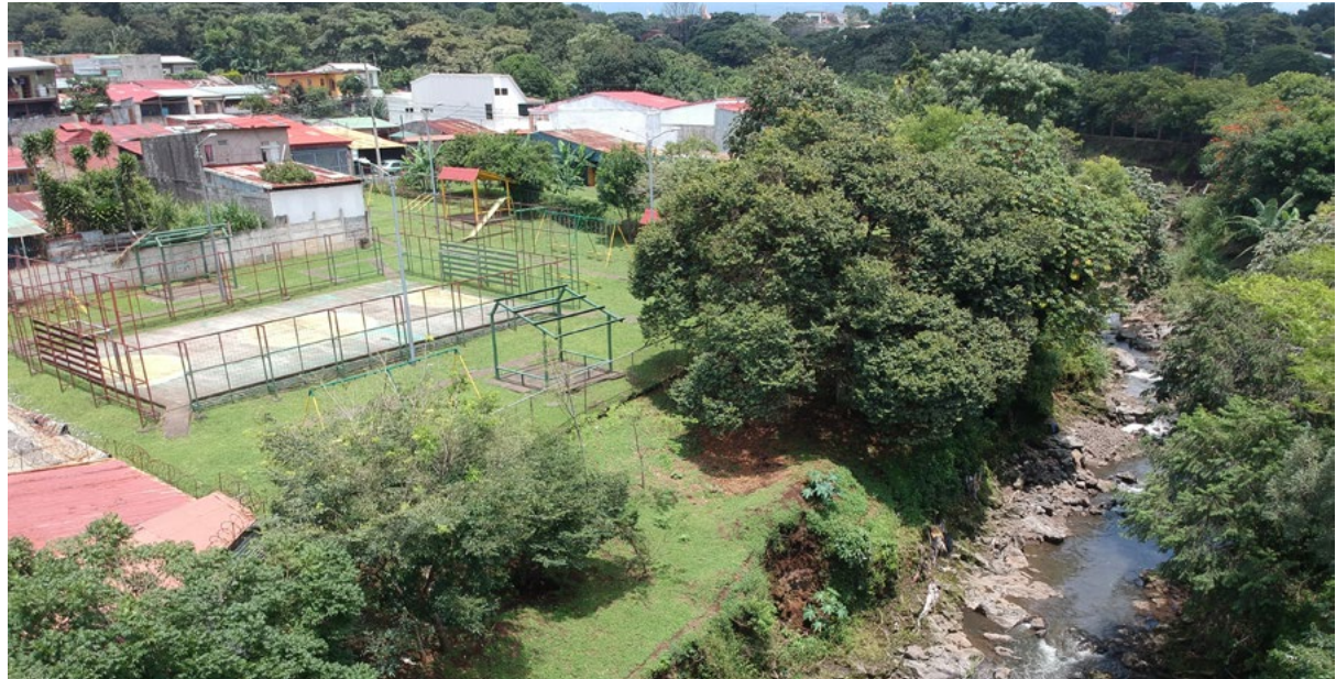
Aerial view of the Quebrada Seca-Río Burío River in Hereda, within the Greater Metropolitan Area of Costa Rica.
