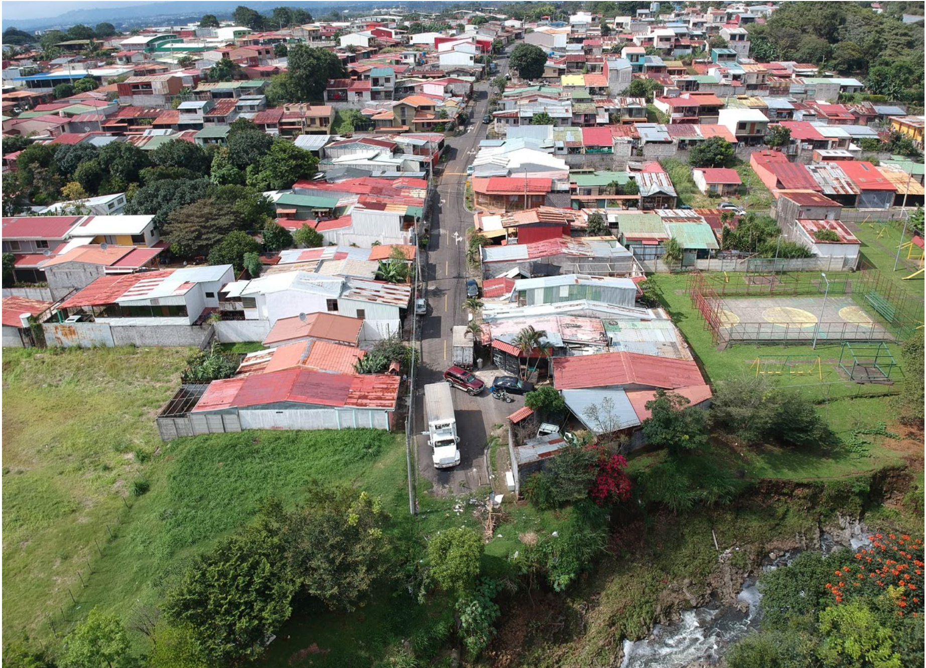
Aerial view of the area of implementation of prototypes in the neighborhood "Siglo XXI" in Llorente, Flores, Costa Rica.
