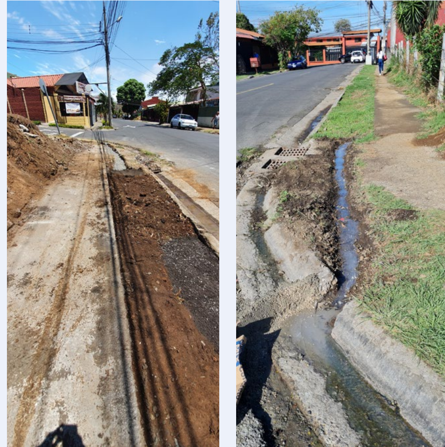
Figure 4.36. Top view of the bioretention area prototype, displaying its condition soon after construction (left) and one year later (right).
