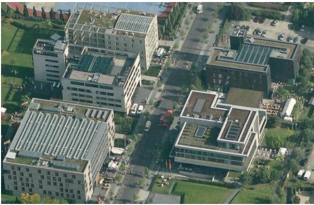
Figure 8. Oblique aerial image of test area "a". The different facade structures, leading to quite heterogeneous PS densities, are clearly visible.
