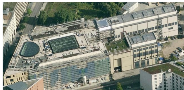
Figure 11. Oblique view aerial image of test area c. The scaffold at the left part of the visible facade indicates construction works and explains the low PS density for this part of the building.
