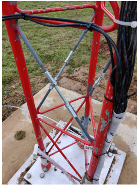
Figure 5.3: Closeup of reversible damage mechanism incorporated into the structure.
