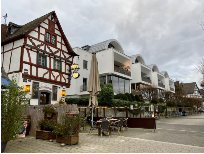
Fig. 6.22 Timber-framed building and the new residential building
