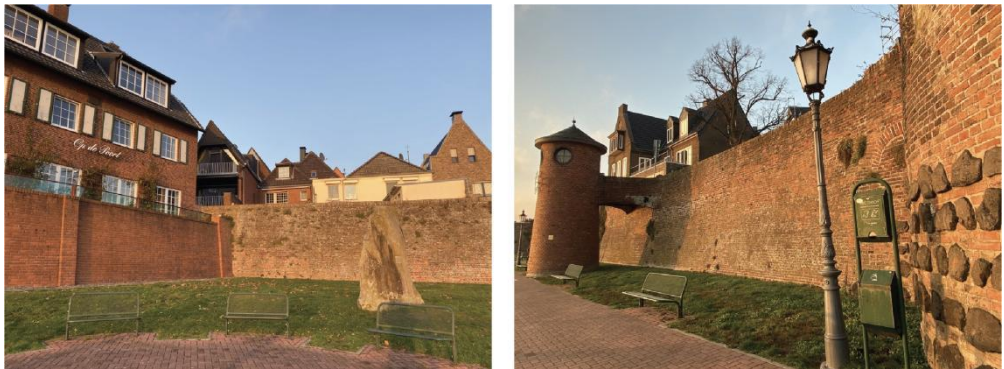
Fig. 6.18 The new wall met the old town wall (left), old wall and the Pegelturm (right)
