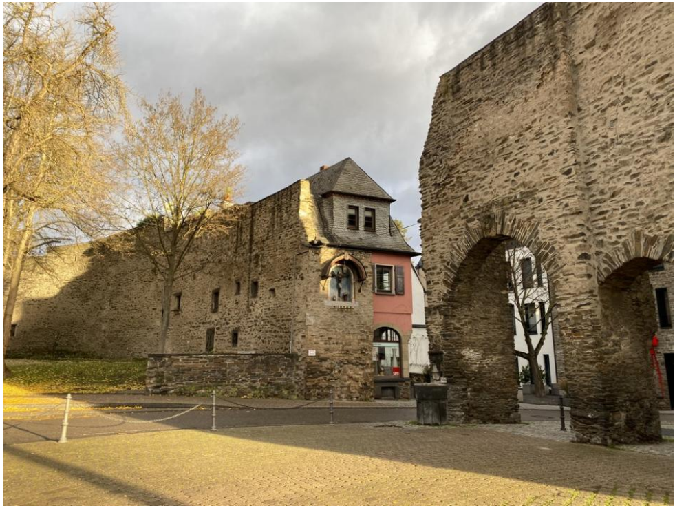
Fig. 6.38 Ancient city wall of Andernach in the morning sun
