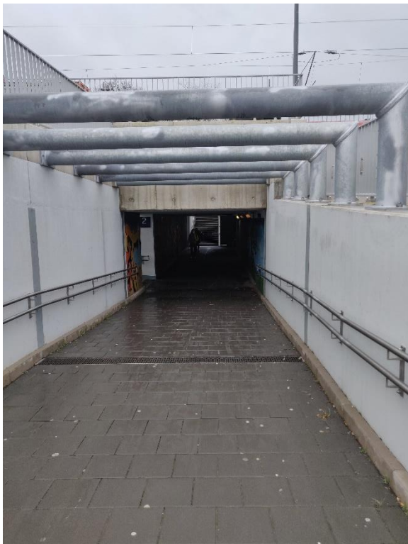
Figure 44: train station underpass end towards Kaufland supermarket by day (own depiction)
