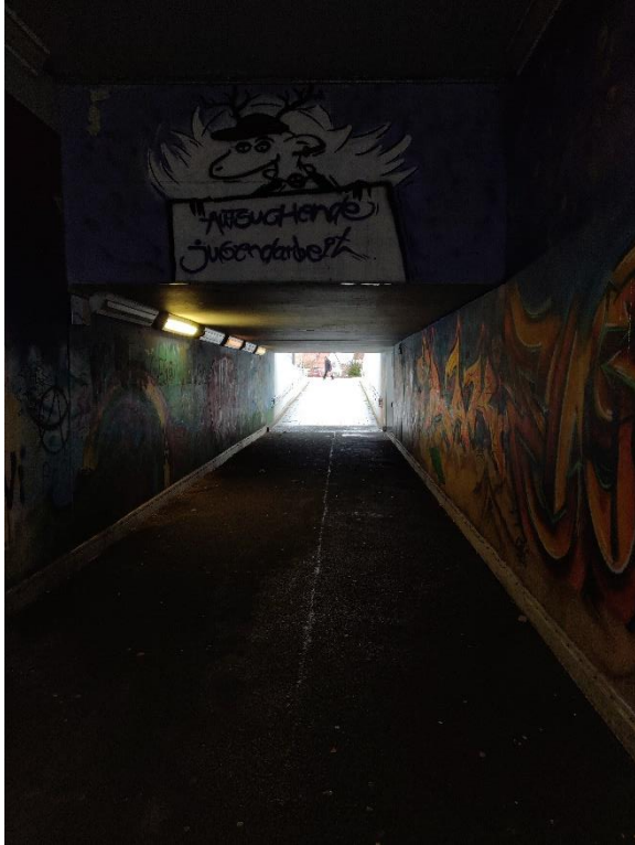
Figure 42: train station underpass by day (own depiction)
