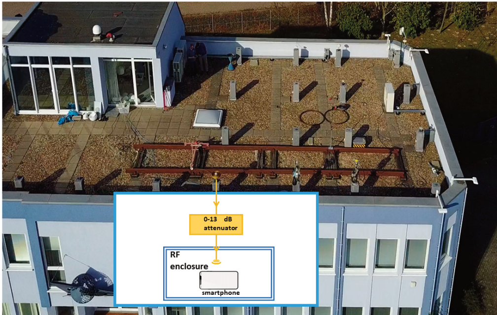
Figure 1. Setup of the experiments carried out in this work. A choke-ring antenna on the roof of the Geo++ GmbH building is connected to a splitter feeding the RF enclosure where the signal is re-transmitted to the smartphone. A 0-13 dB attenuator was applied to the signal re-transmitted to the smartphone. The pillars on the roof were used to collect open-sky data.
