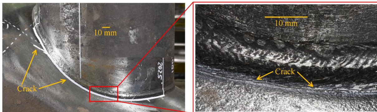
Figure 7. Exemplary crack path after through thickness cracking
