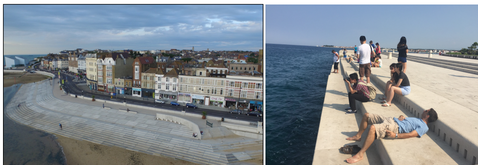
Figure 1.1: Examples of stepped revetments: (a) Stepped revetment providing access to the beach in Margate, United Kingdom. Photo by Dean Barkley. (b) Promenade in Zadar, Croatia
