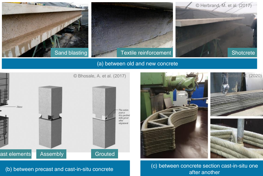
Figure 1.1 Practical applications of concrete interface in constructions: (a) between old and new concrete for rehabilitation [2]; (b) between precast and cast-in-situ concrete in modular construction [3]; and (c) between concrete section cast-in-situ one after another [4]
