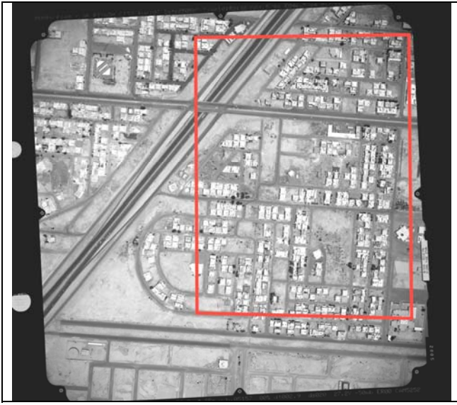
Figure 32: Area used for following building monitoring marked by red line
