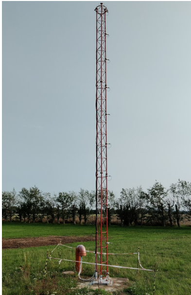
Figure 24: Photograph of girder mast structure.
