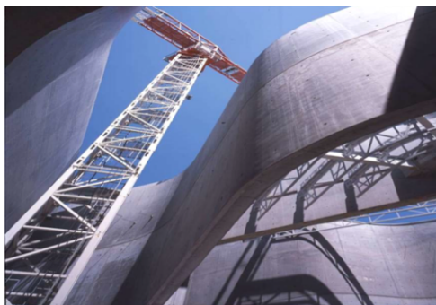
Figure 2.4: Joint-less walls of the MAXXI in Rome (Troli and Colleparidi, 2011)
