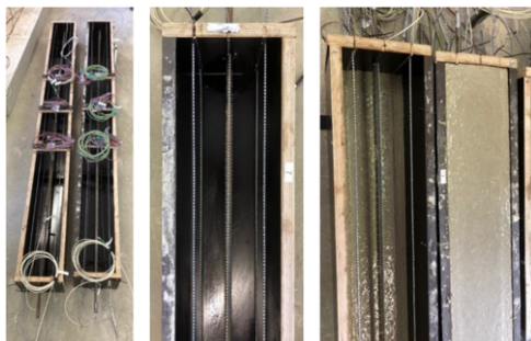
Figure 4.10: Concreting of beams and the measuring equipment installed in formwork
