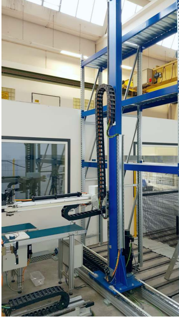
Fig. 2. Experimental testbed stacker crane
