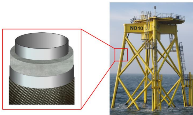
Figure 1. The foundations of offshore (mega) structures account for a significant proportion of the total weight of the structure. Transporting the foundation structure is a logistical challenge. Weight can be saved on strut-shaped components by replacing steel cross-sections with concrete cross-sections.
