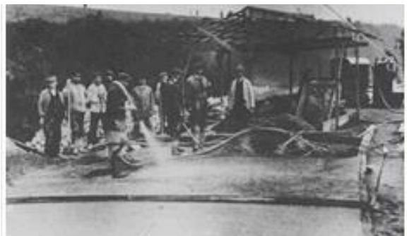
Figure 1: „Torkretieren“ of a road in 1926 [Torkret GmbH]
