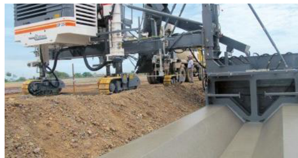
Figure 3: Slip forming of rain water drainage [5]
