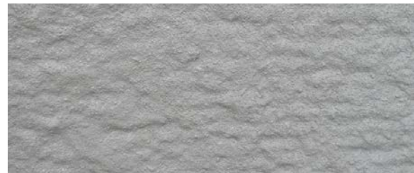
Figure 10: Surface structure of the dried shotcrete
