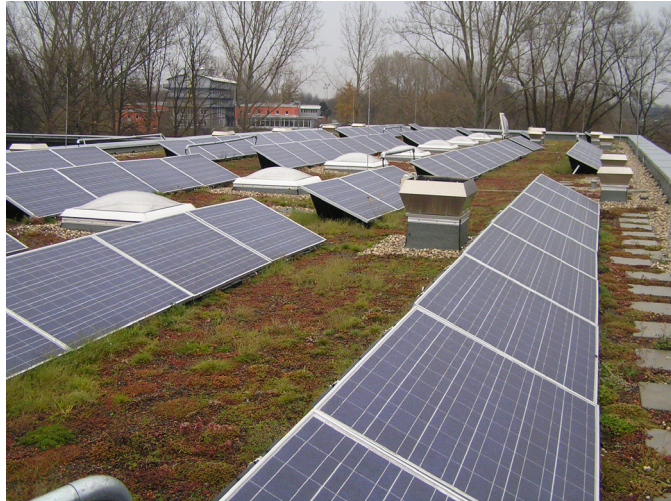
Fig. 3. On the roof of the maintenance depot Stammestraße a photovoltaic system was installed in addition to the roof greening. (DEPARTMENT ENVIRONMENT AND URBAN GREENSPACE, STATE CAPITAL HANNOVER)
