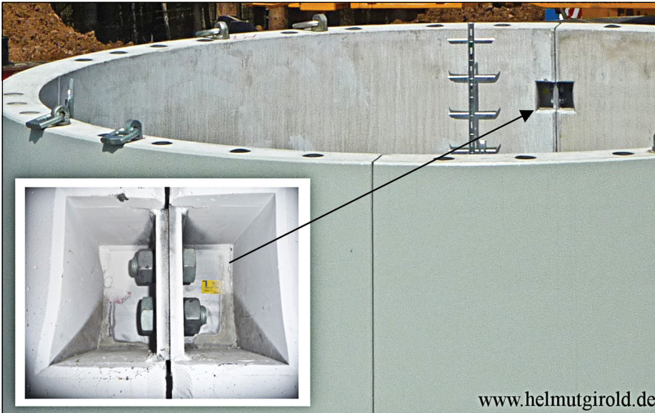
Figure 4 Bolted connection of two precast concrete segments
