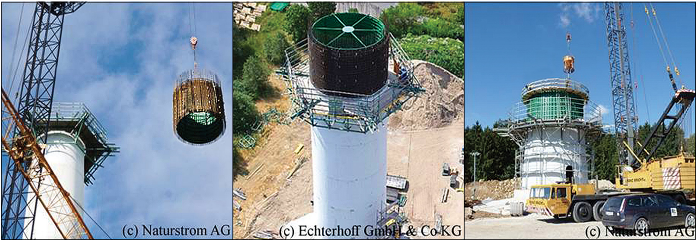
Figure 1 Climbing formwork of a cast-in-place wind tower
