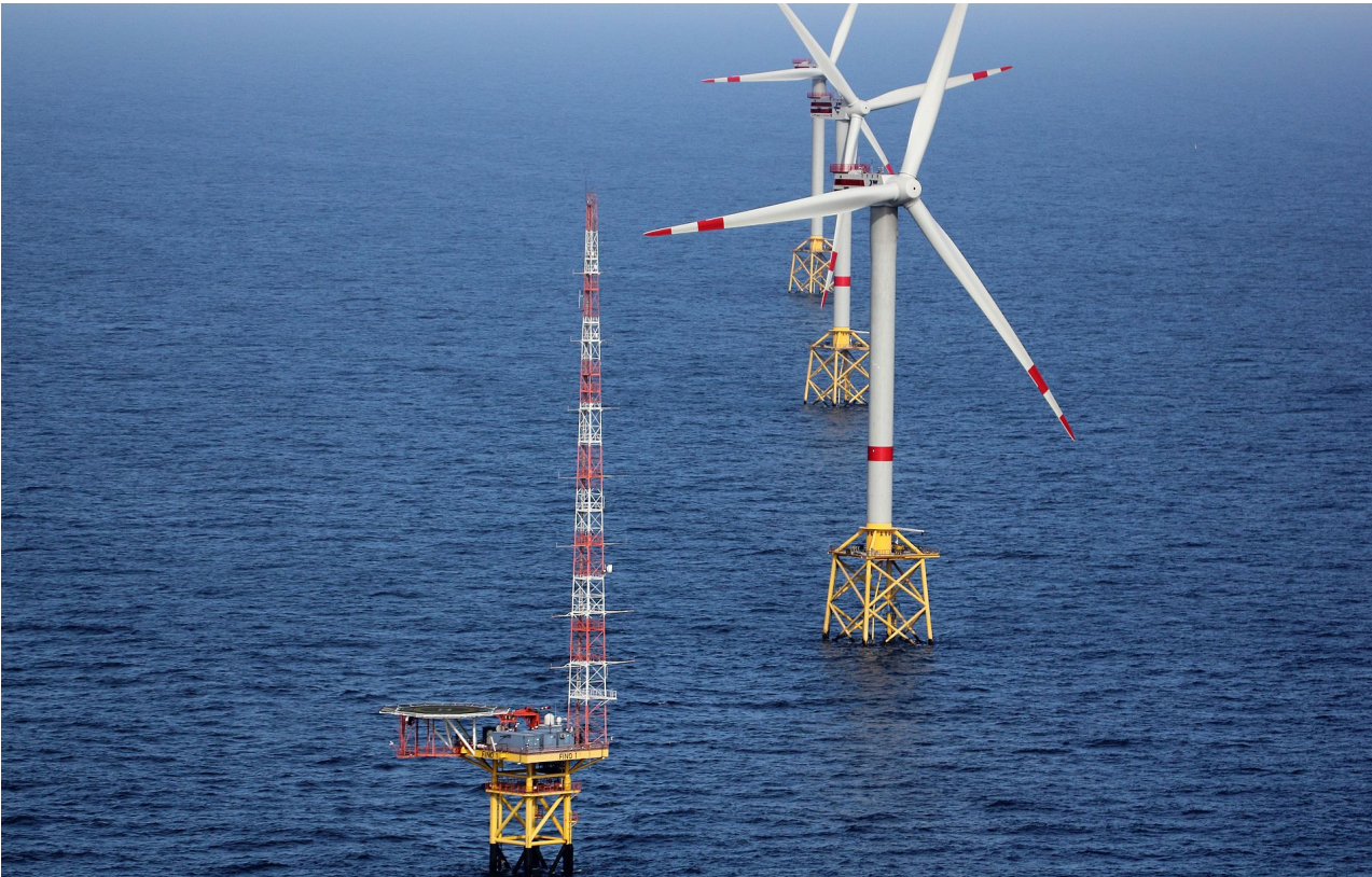
Figure 1.1: Three REpower 5M offshore turbines with jacket substructures in the offshore wind farm alpha ventus, research platform FINO1 in the foreground (Rademacher 2012).
