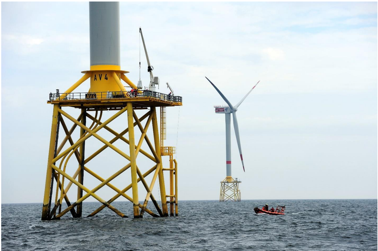
Figure 1.1: Two offshore wind turbines with jacket substructure located at the German offshore wind farm alpha ventus (© DOTI 2011 / alpha ventus, Photo: Matthias Ibeler)
