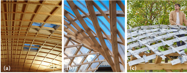
Fig. 2. Various types of gridshells fabricated by bending straight lamellas. (a) The Polydôme by Julius Natterer using stacked geodesic planks, and a diagonal geodesic cover [Natterer et al. 2000]; (b) Timber gridshell by Eike Schling et al. combining asymptotic and geodesic lamellas in a trihex grid ( https://eikeschling.com ). (c) Pseudo-geodesic gridshell by [Mesnil and Baverel 2023], using inclined strips.
