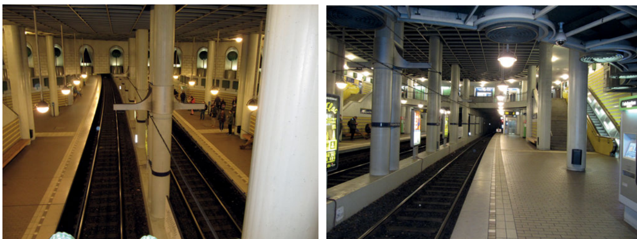
Figure 3: Grid representation of the Königsworther Platz subway station in a perspective view (above) and in horizontal and vertical cross sections (middle). Only the central part of the simulation area is shown. Pictures of the real station are given below.
