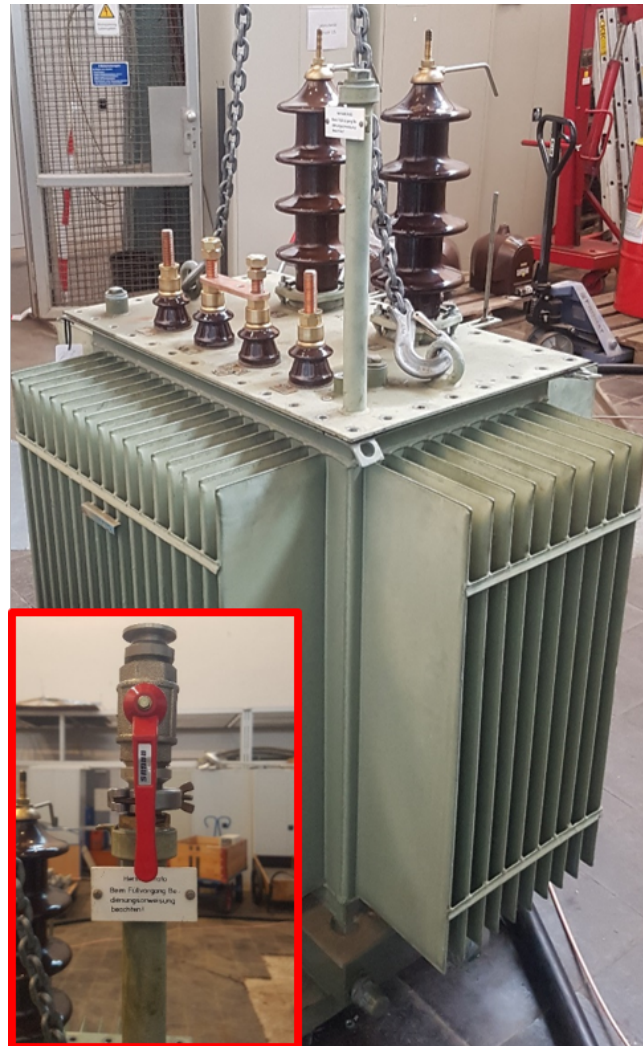
Figure 2.19: Hermetically sealed railway transformer and its oil filling pipe
