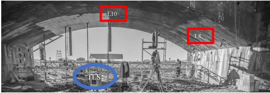
Fig. 3 A bridge under load: localization of the points L10 and L8
